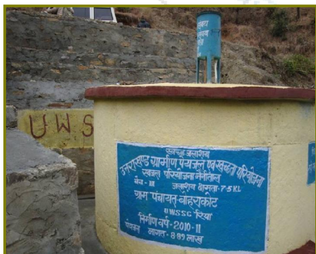
CWR & chlorinator of a W/S scheme Riva. GP Boharakot
